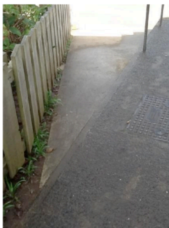
Ramp for change in levels tapered and narrow – tipping risk.
