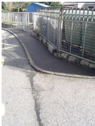
Front access path and pavement – narrow and no tactile paving.
